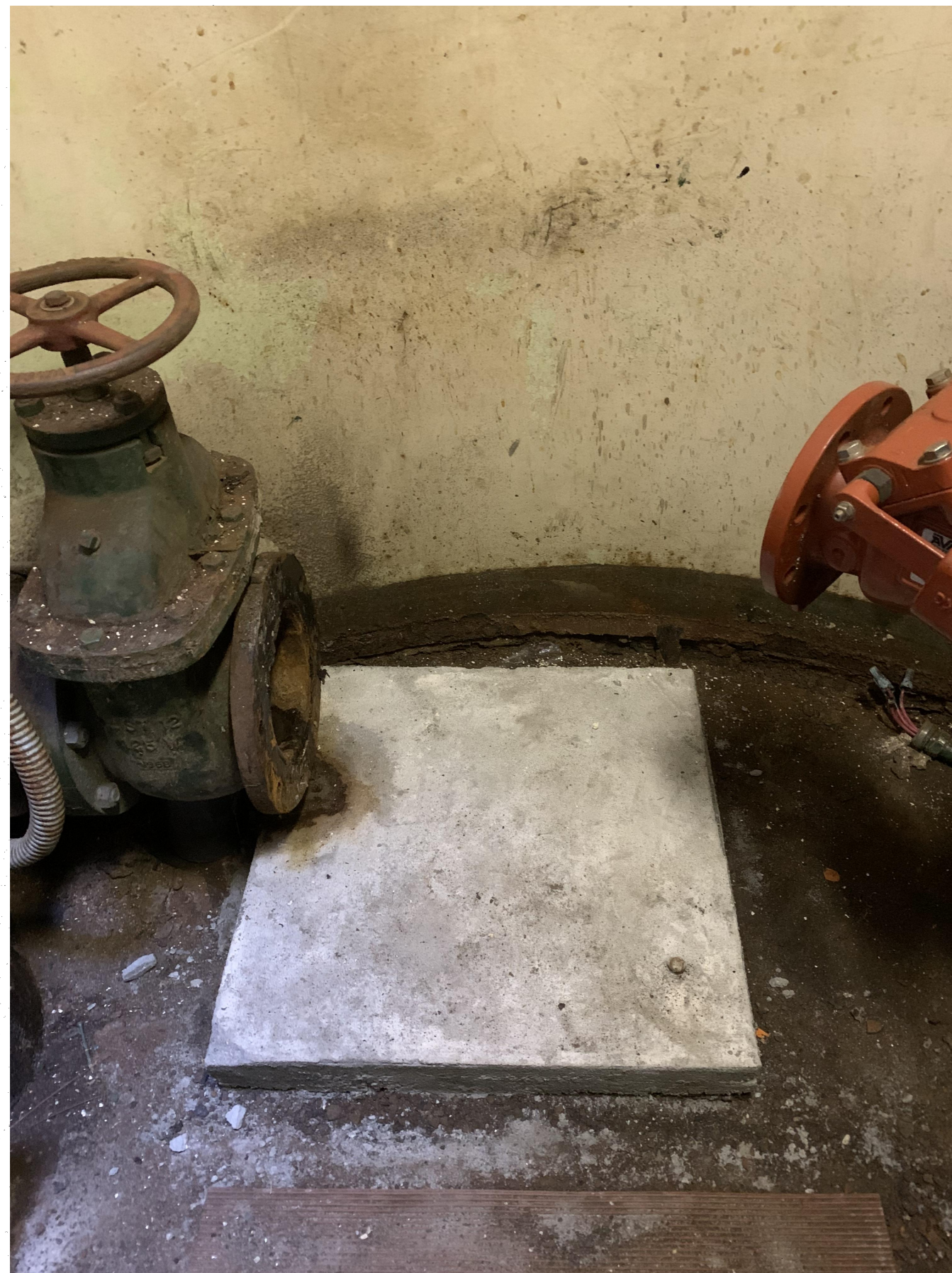
Existing New Pad for Pump #1
