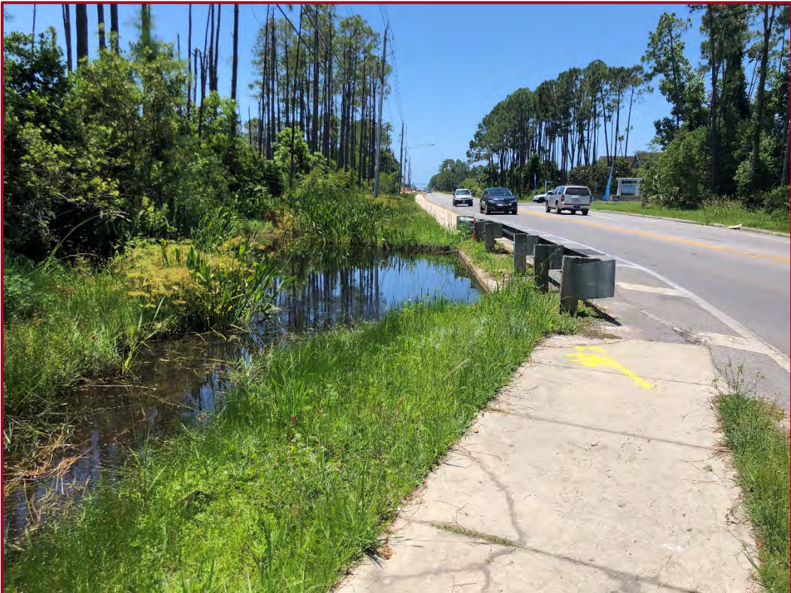
FIGURE 3B: EXISTING SITE CONDITIONS NEAR STATION 736+60 (FACING NORTHEAST)
